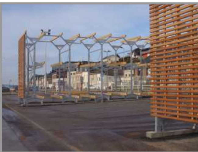
RACKUP 3 stages with wood siding Pictures taken from the dry stack of Fécamp at the end of the construction.
